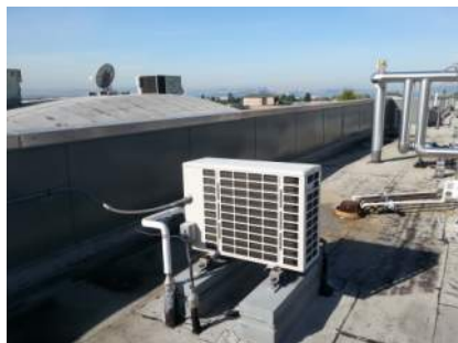
Condensing Unit for Split System
