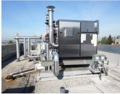
Roof Mounted Condensing Boilers
