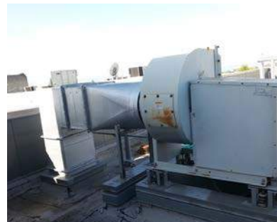
Building Toilet Exhaust Fan
