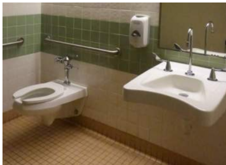
Existing Toilet and Lavatory
